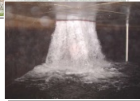
Water cascades into C2 Reservoir after passing through the turbine.†
