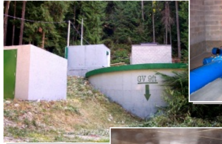
Service Reservoir and Powerhouse*
