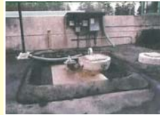
Enclosed and automated septage receiving station with downstream dilution tank
