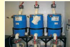
Activated Carbon Odour Control
