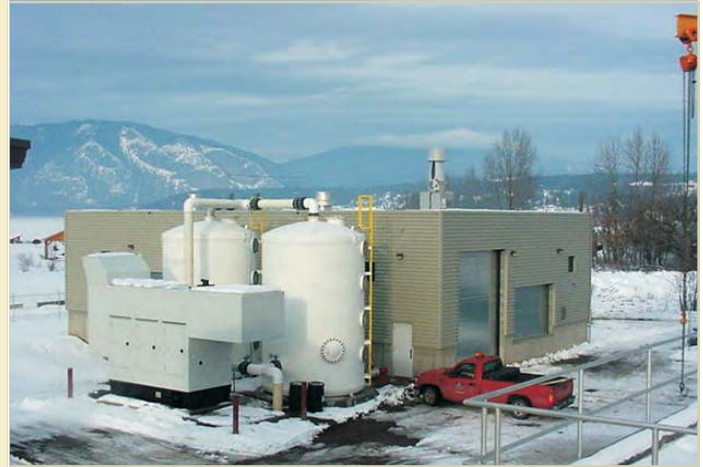
Biological Scrubber Towers, Ozone Odour Treatment & Wet Chemical Scrubbers City of Salmon Arm, British Columbia
