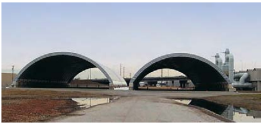
Secondary Biofilter Odour Control System Greater Vancouver Regional District Annacis Island Wastewater Treatment Plant, Delta, B.C.
