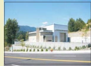
David Avenue Pump Station City of Coquitlam, B.C.
