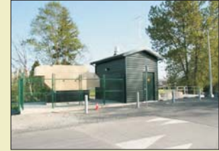
Carter Street Storm Pump Station City of New Westminster, B.C.
