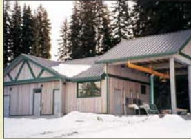
Sanitary Pump Station Resort Municipality of Whistler, B.C.
