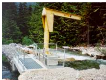
Greeley Creek intake structure
