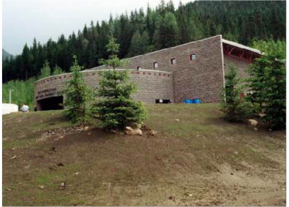
Greeley Creek Water Treatment Plant
