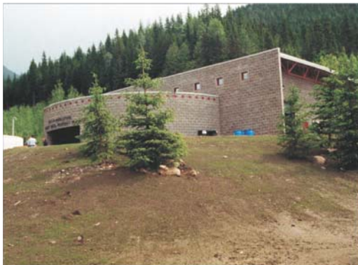
Greeley Creek Water Treatment Plant
