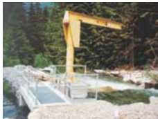
Greeley Creek intake structure
