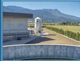
Main Plant Scrubber
