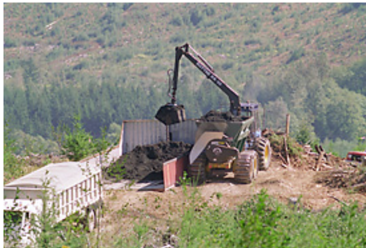
King County, Seattle, WA, Loading Flinger with Dewatered Biosolids from Portable Bunker
