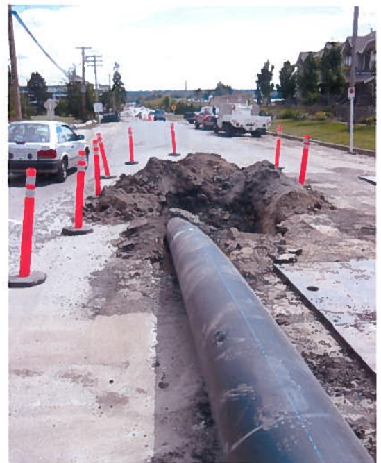
The new HDPE forcemain being pulling into pit at 67th Avenue.
