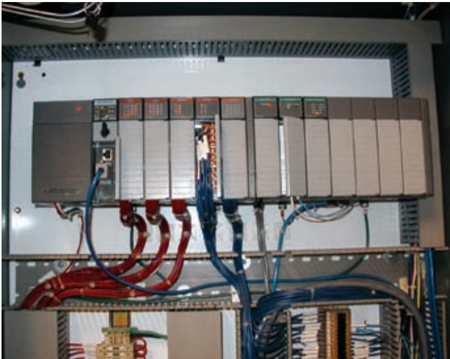
PLC controller at typical SCADA facility used for local control and communications
