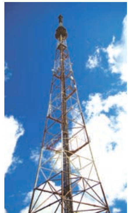
A typical radio communications tower
