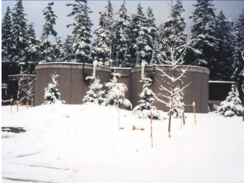
Figure 18 - Resort Municipality of Whistler WWTP ATAD Venturi-Pump
