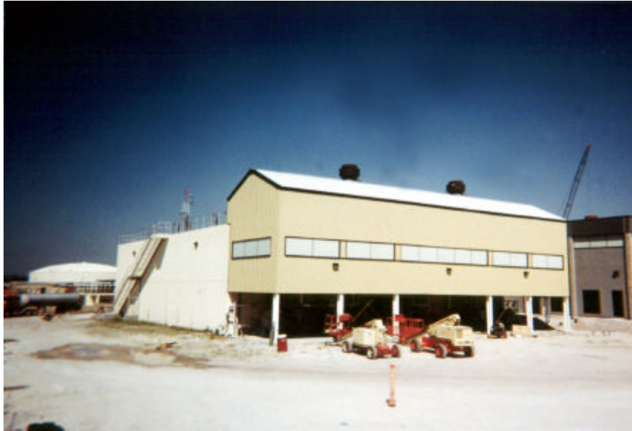
Figure 8 - City of Sunrise, Florida, Sawgrass WWTP ATAD
