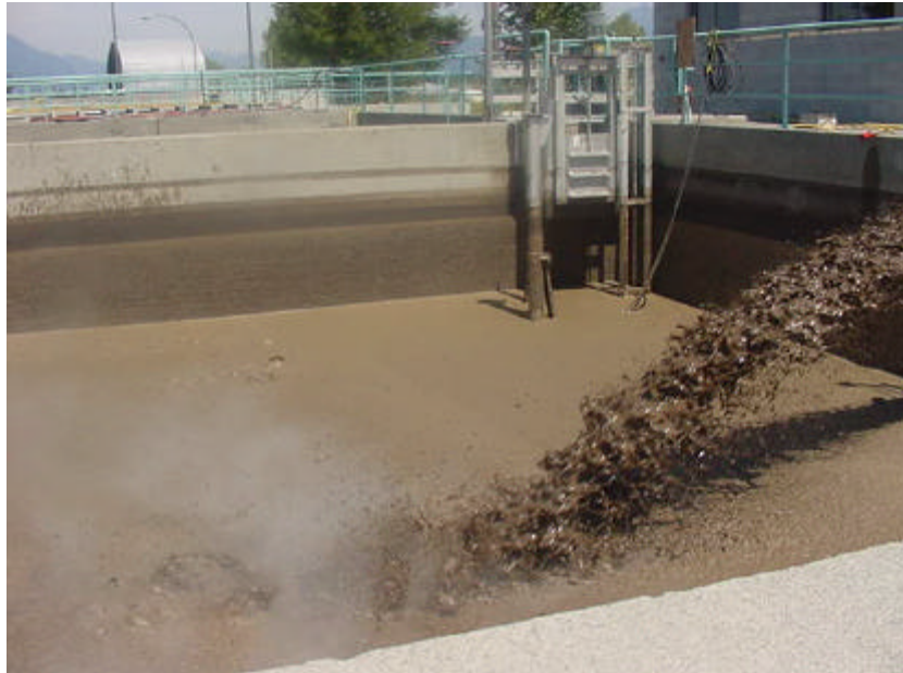
Figure 7 - NW Langley, B.C. WWTP Pump Foam Reduction on Timer
