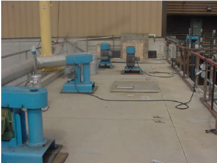
Figure 5 - District of Salmon Arm, B.C., WPCP ATAD Turborator Aerator Mixers
