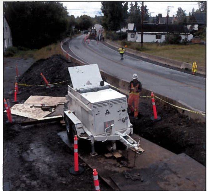
The existing main ran under the shoulder.
