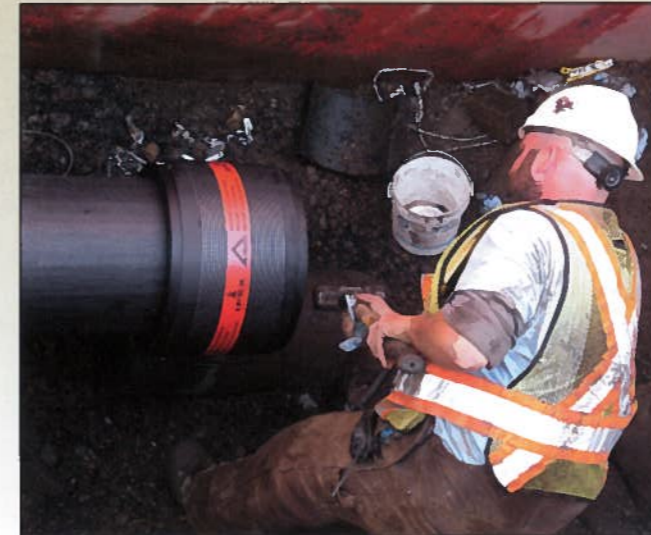
The new sections of HDPE main were joined using electro-fusion couplings.
