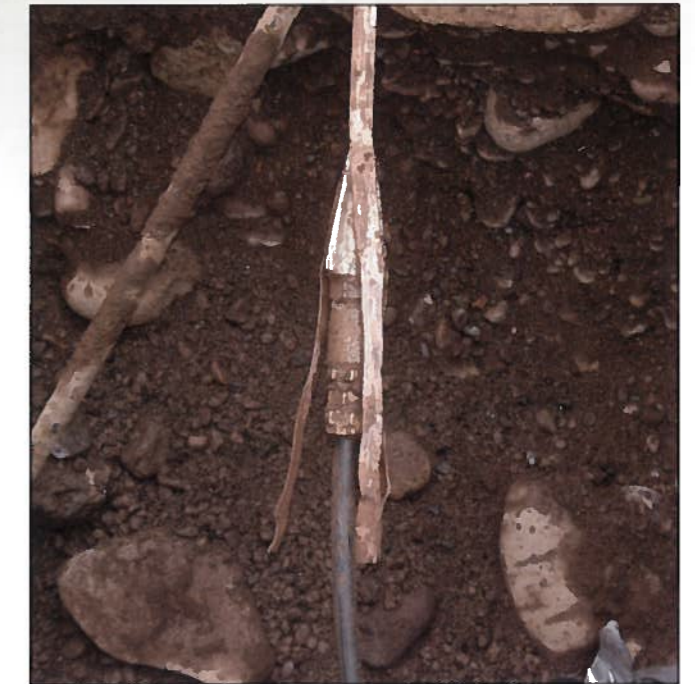
Service connections under the highway were replaced using a static burster.
